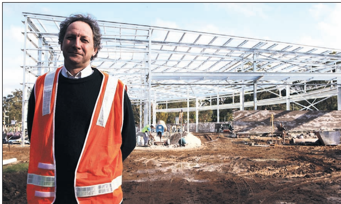
Big upgrade: Richard Mulvaney in front of the workshop construction site.
